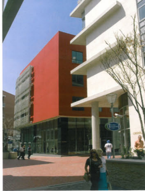
The intersection of Cross and Slip Streets.
