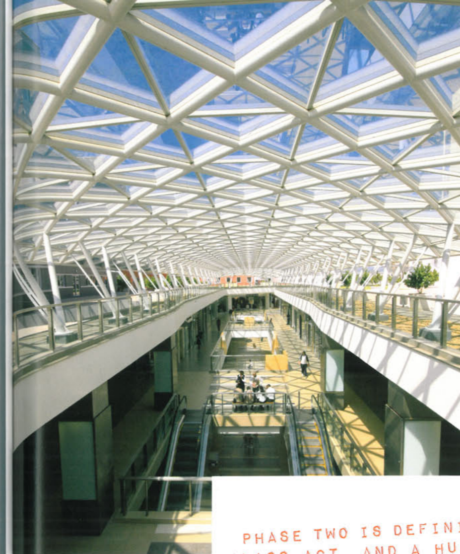
The award-winning Galleria roof lets in light and air, thus maintaining the outdoor feel of the precinct while allowing for rainy day shopping.
